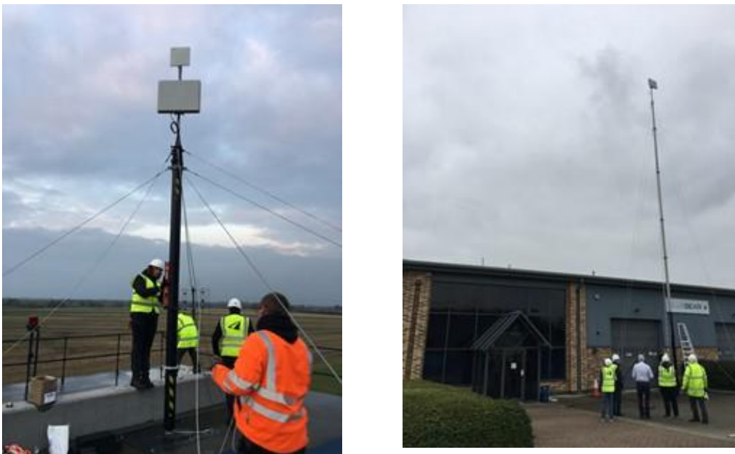
Figure 1: Installation of the masts at Blue Bear offices and Twinwoods
